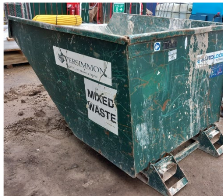
Auto-locking skip, no catch/ rings or chains needed
